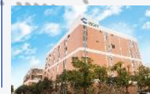
GMP Facility (Jinshan)
